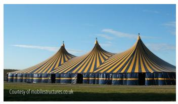
Fig. 4 - MT66 series 'palisade' tent, note that the three in-line 'king-poles' precludes using this structure for anything other than dance/rave events
